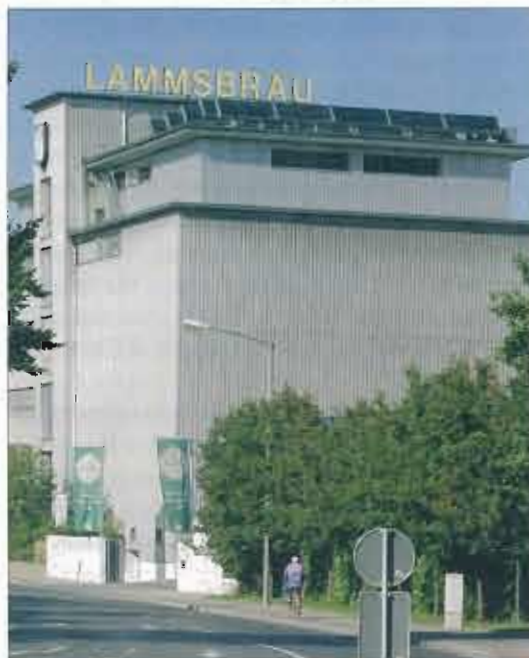
72.5 m 2 of air collectors are installed on this brewery in Neumarkt, Germany. Per hour, up to 5,500 m 3 of air is heated by solar energy, equivalent to a thermal nominal output of 48 kW.
