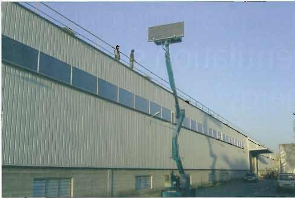
Technicians install air collectors on one of automotive supplier Palmela S.A.'s warehouses in the eponymous city in Portugal.
